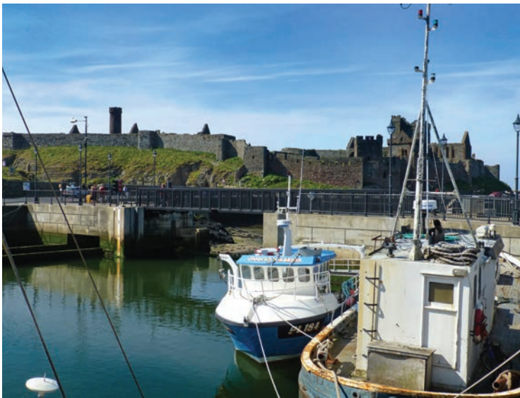
Peel Harbour swing bridge | Isle of Man
