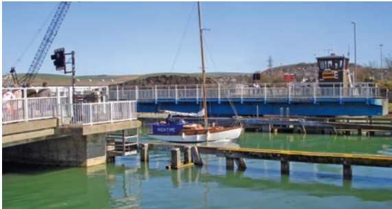
Newhaven swing bridge | East Sussex, England
